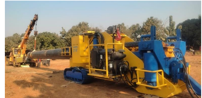
Slurry Pipeline: Bending Pre-Qualification Trial
